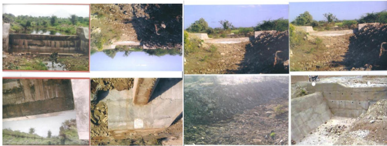
Check Dams Constructed by BSST
